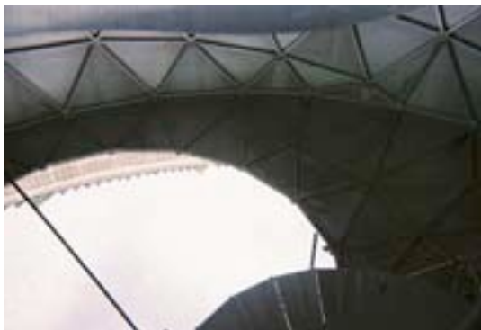
Primary dish, a piece of the secondary at the top, and a piece of tertiary lower right.
